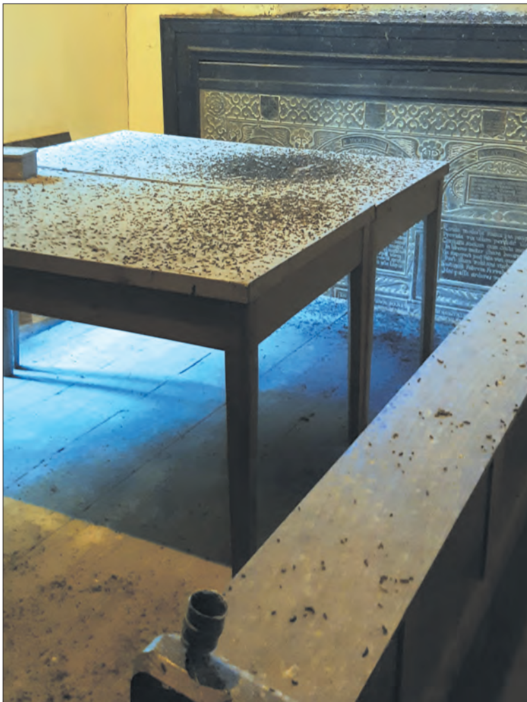
Fig. 2: Extensive bat droppings and urine staining at St Moren's, Lamorran, Cornwall. (Bats in Churches)
