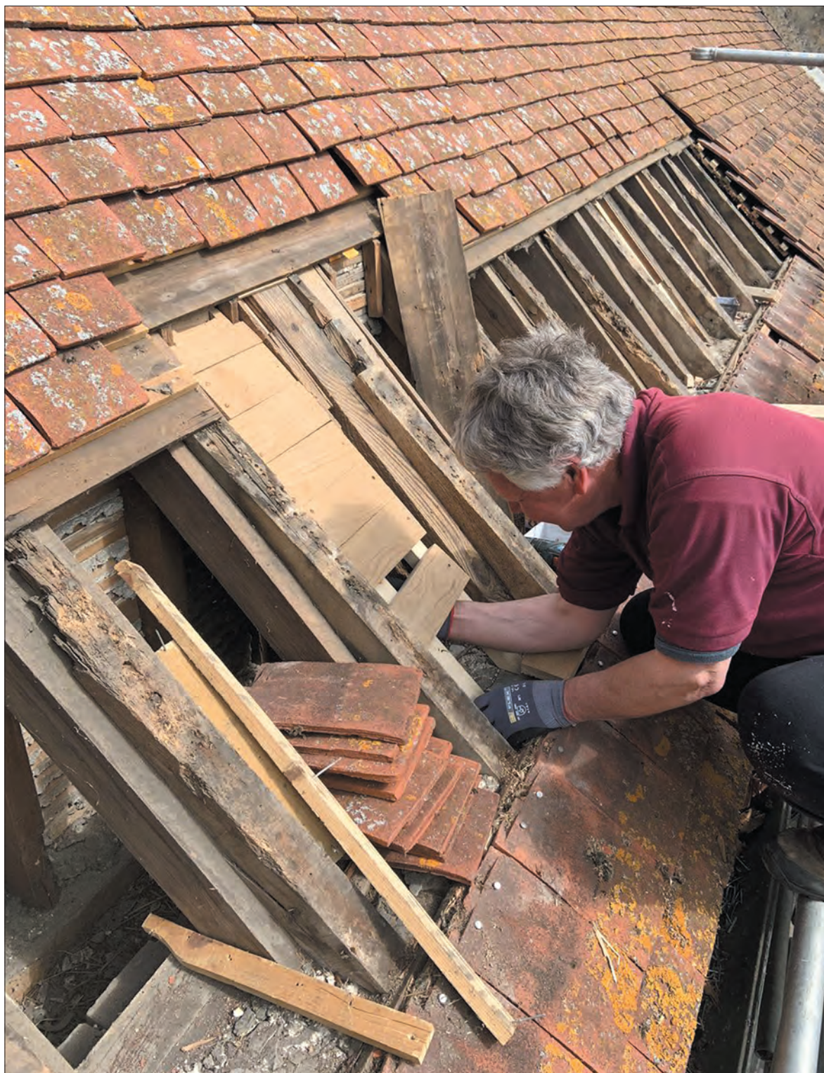
Fig. 6: A bat box being installed in the roof of All Saints', Swanton Morley, Norfolk. (Copyright: Dr Lotty Packman Wild Wings Ecology)
