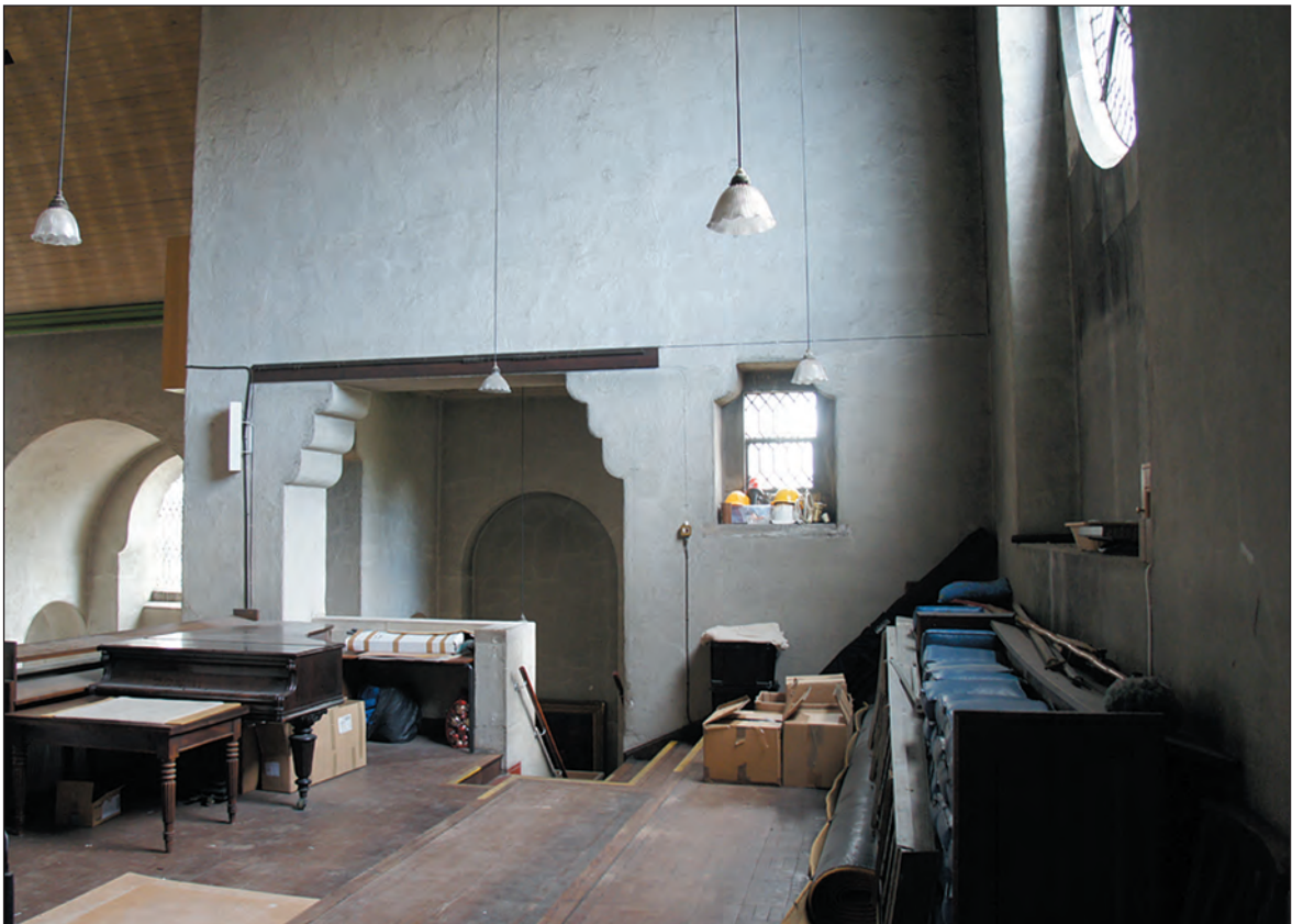
Fig. 6 The West Gallery of St Francis, Bournemouth with its almost Art Deco shouldered openings; note also the original 'Atlas White' cement walls. (Photo: Alwyn Ladell)
