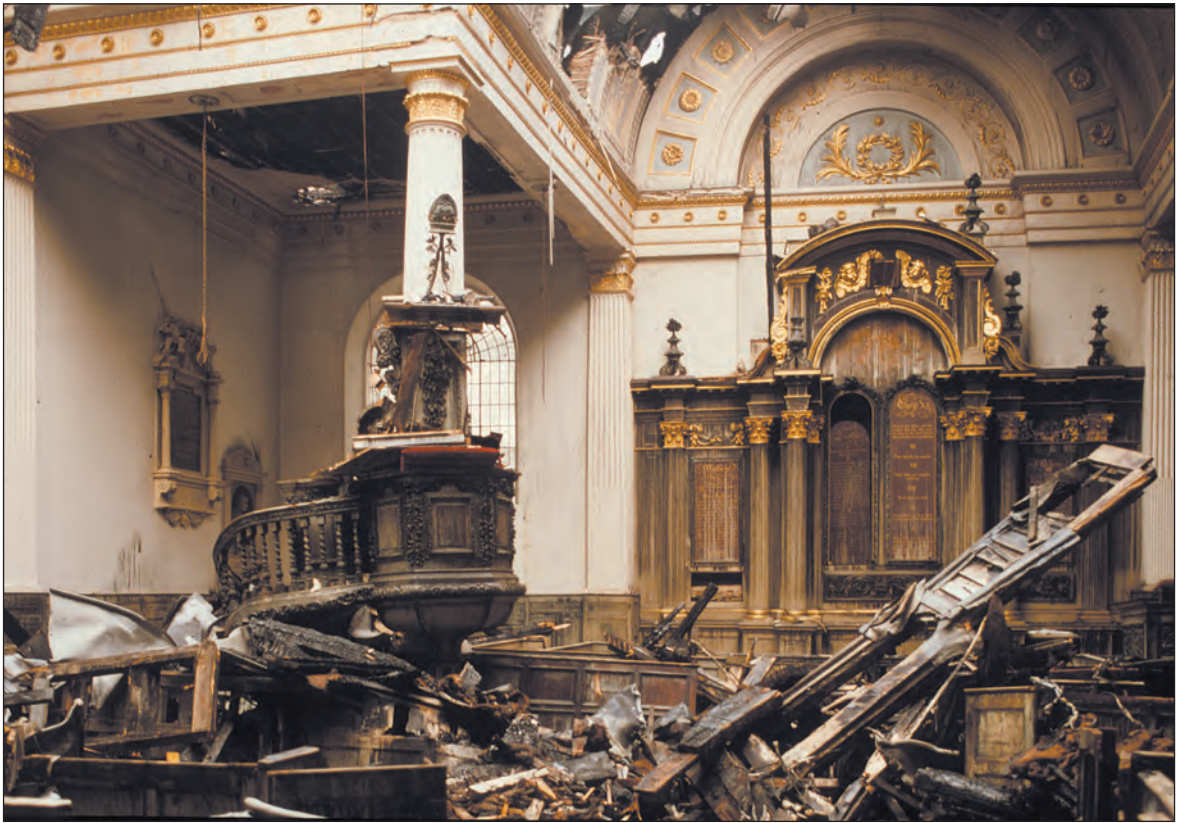
Fig. 3. The interior of the church on 12 May 1988, two days after the fire that destroyed most of the roof: the pulpit and reredos had been damaged but had not been burned.
