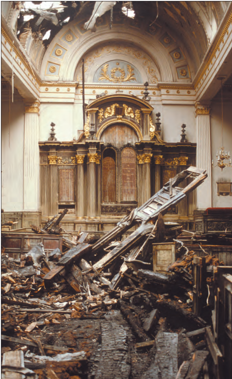
Fig. 7. The east end of St Mary-at-Hill on 12 May 1988: many but by no means all of the box pews had been smashed by falling timbers from the burning roof. (Photo: Gavin Stamp)
